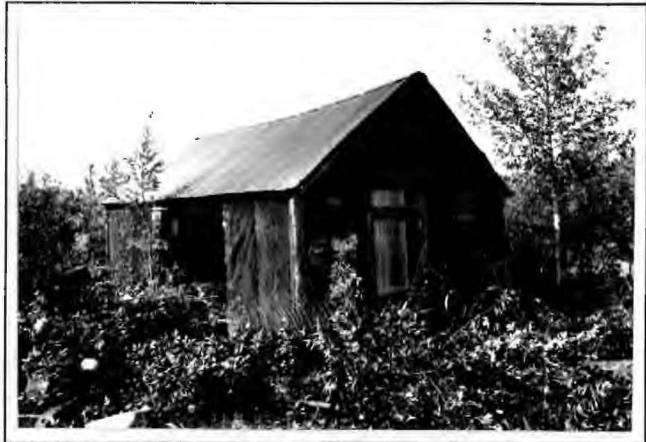
Figure 59. The NADC Parts Warehouse, 1993. The view is looking northwest.
